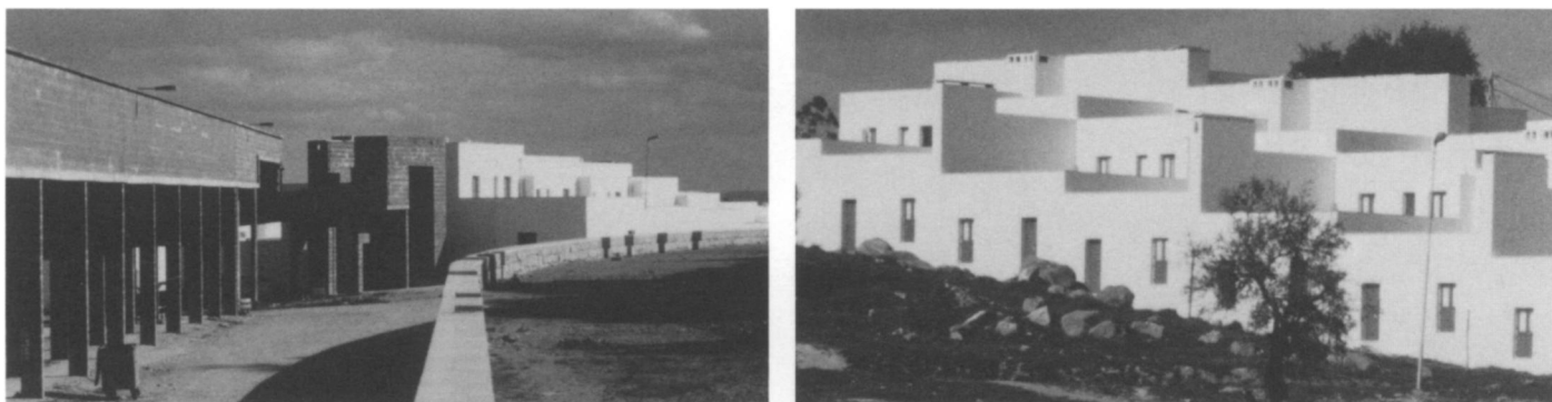
Alvaro Siza Vieira, Quinta da Malagueira housing, Evora, Portugal, 1977–to date
